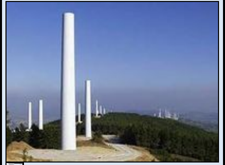
Fig 8(a) Tubular tower
