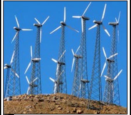
Fig 8(b) Lattice tower
