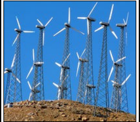
Fig 8(b) Lattice tower
