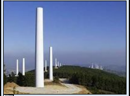
Fig 8(a) Tubular tower
